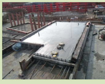
PRE-CAST WALL AND BEAM
