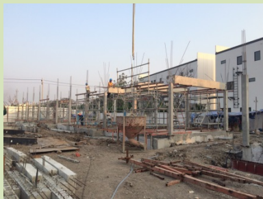
Pre-Cast Beam level 2
