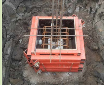
PILE CUT-OFF AND PILE CAPS
